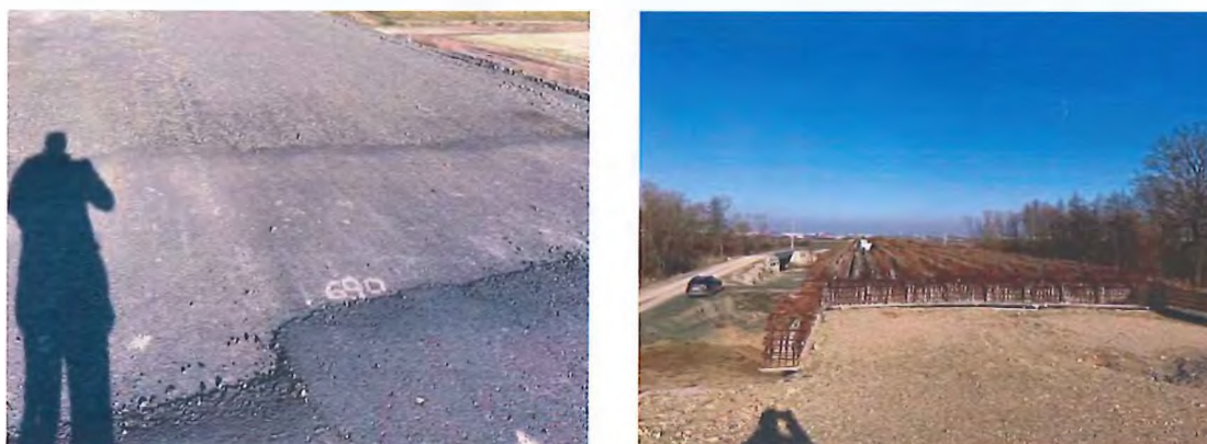
Fig. 6.5.33-3 Pod peste Bega: rampa sud
